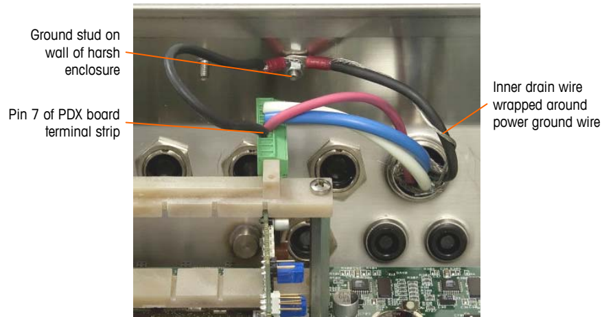
Figure 2-47: PDX Home Run Power Ground Connection, Harsh
